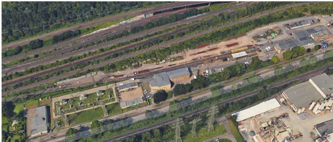
Outdoor facilities of the German Railway (DB – Deutsche Bahn)
